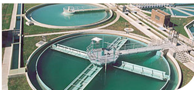
Water and waste water treatment
